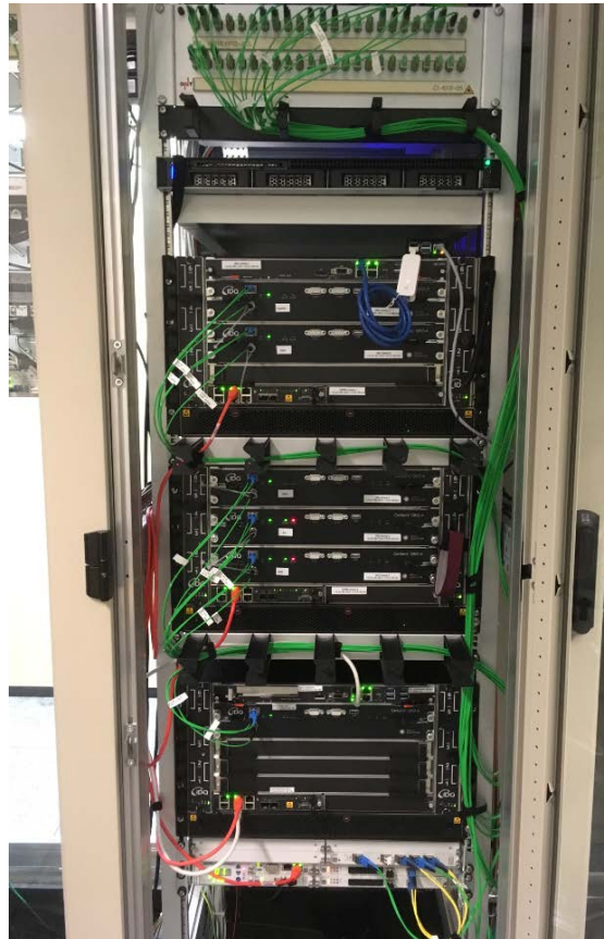
QKD device and encryptors installed at SIG Headquarter
